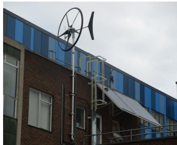
1.5 kW HWT and 1 kW PV system
