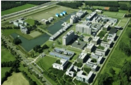
Software development center at high-tech campus, Eindhoven, the Netherlands
