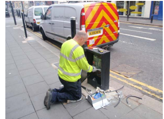
Charging point installation on Clayton Street
